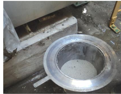
Fig. 4 molecular sieve particles in the strainer.
