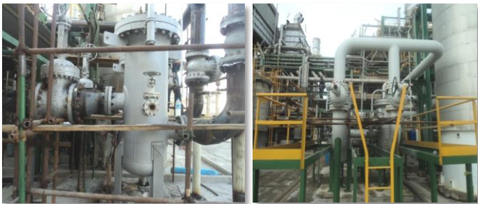
Fig8. Filters after installation
